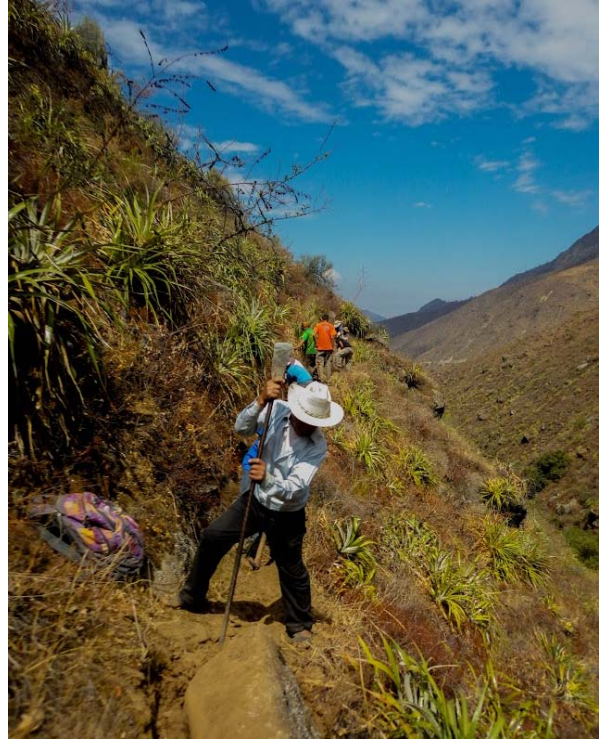
Trenching the 3.5 km long pipeline
