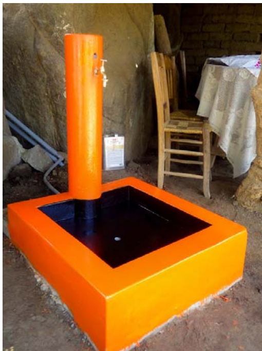
A finished tapstand
