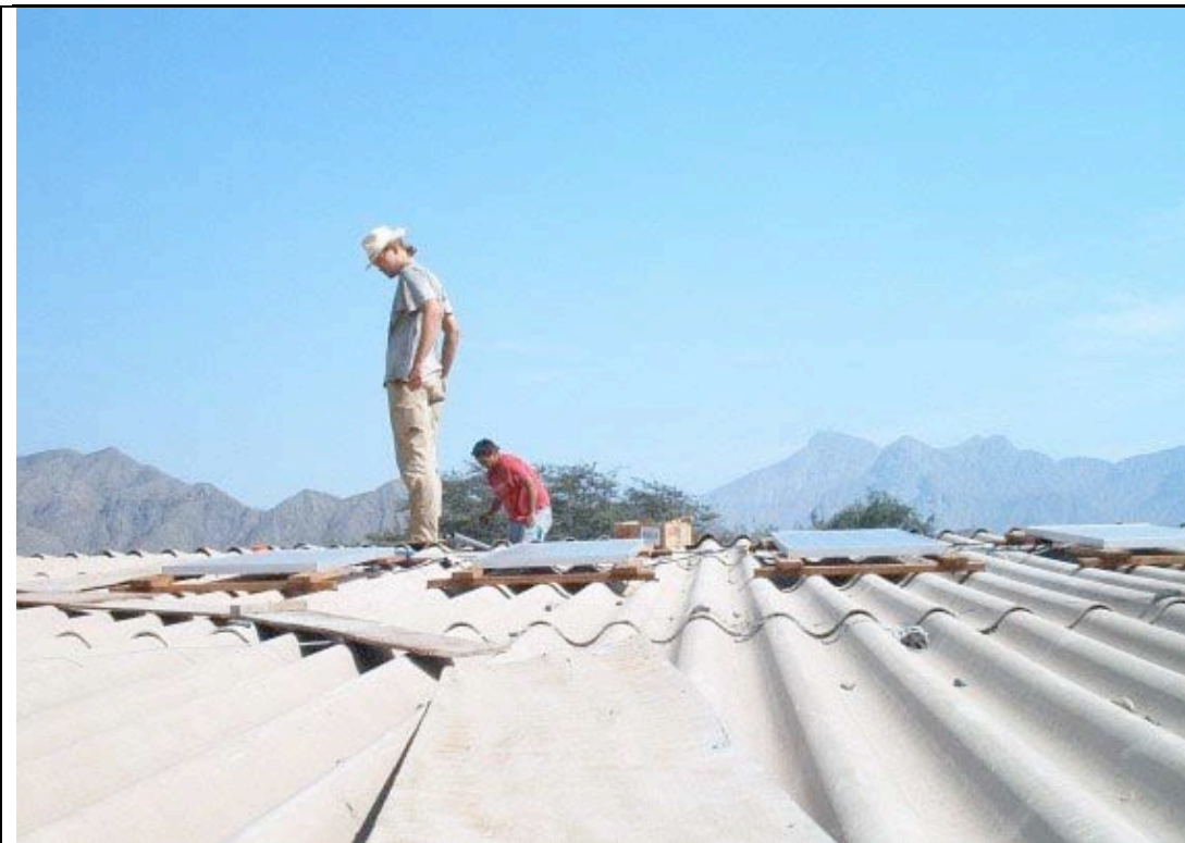
Image of Princeton engineers installing solar panels on school building
